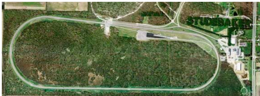
An aerial view showing the trees planted in the upper right hand corner to spell Studebaker.
